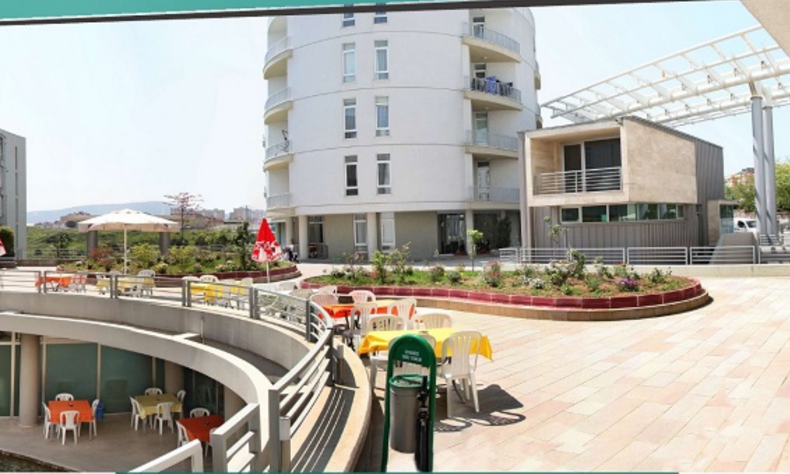
Oval Bahçe Sitesi 264 Daireli Konut Oval Bahçe Compound 264 Residential Units Sancaktepe / İstanbul 2010
